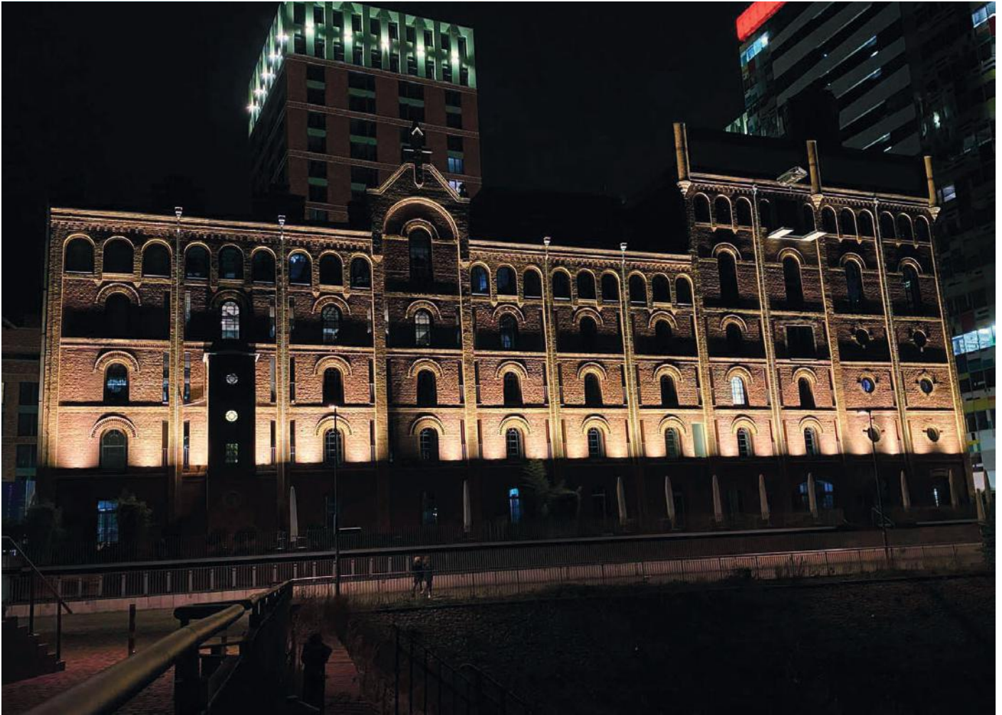
Old malt house, Düsseldorf, Germany ©Hoffmeister; Luminaire: SILL 02M
