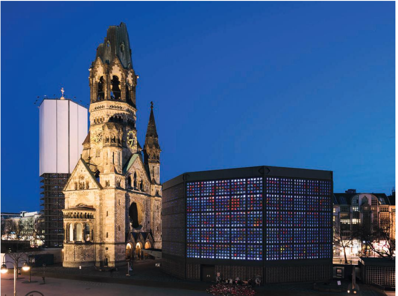
Kaiser Wilhelm Memorial Church, Berlin, Germany. Luminaire: 49. Light planning: Kardorff Ingenieure Lichtplanung GmbH ©Linus Lintner
