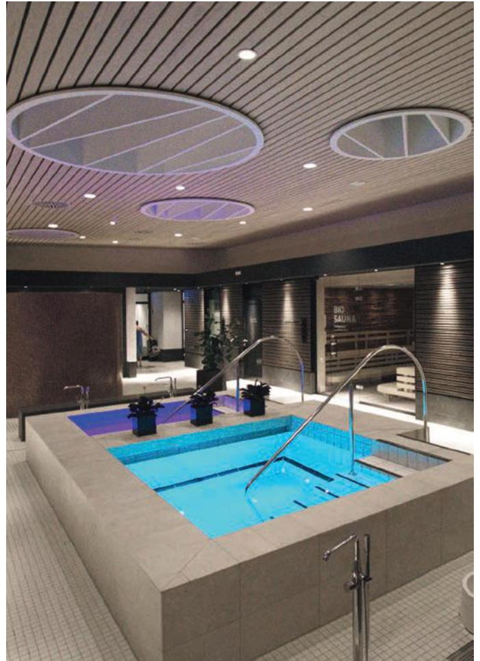
Fresch Swimming pool Freising, Germany. Architects: Venneberg & Zech. Electrical design: Mr. Methling, Ibah ©Hoffmeister; Luminaire: complx.100
