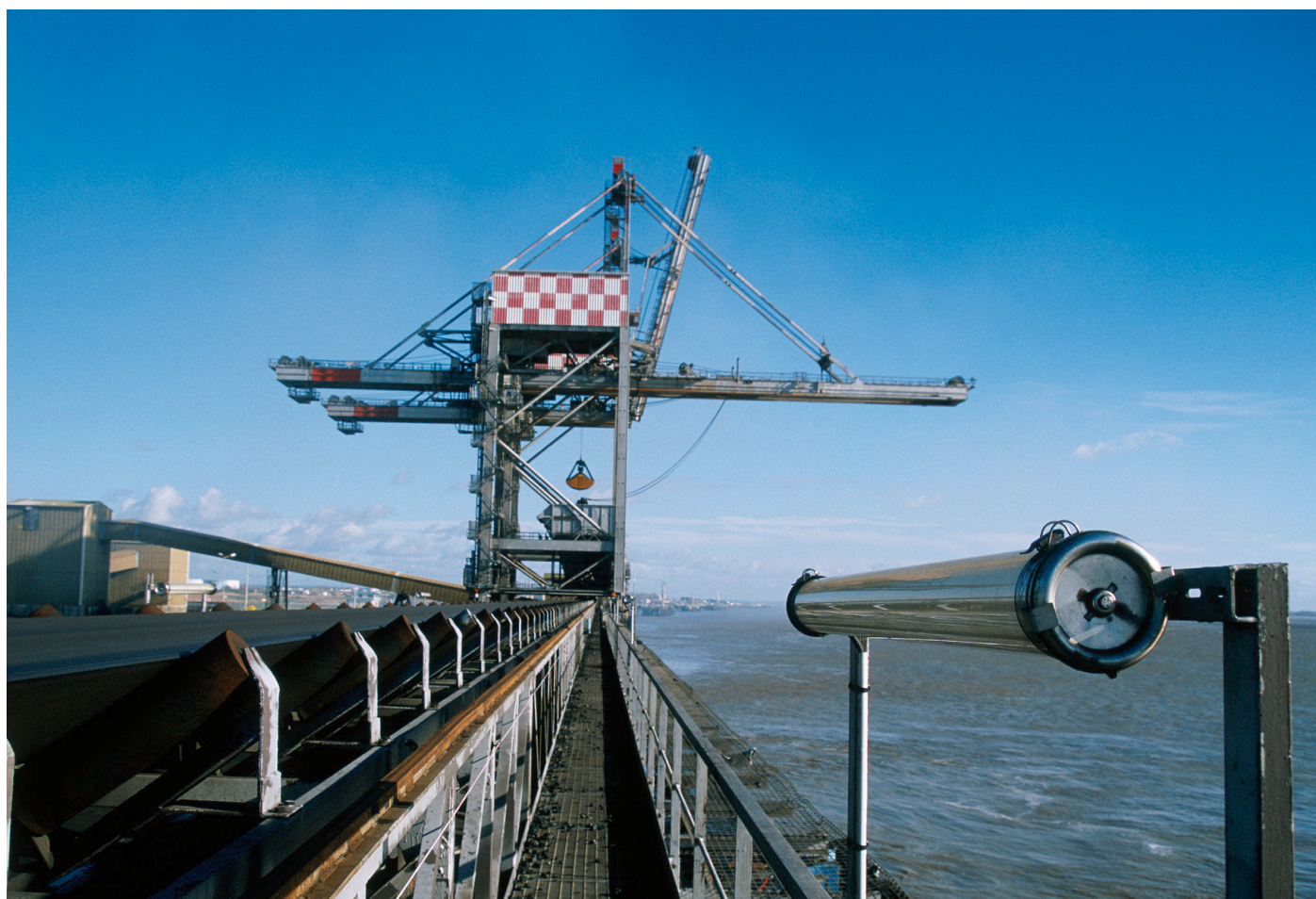
Port of Nantes Saint-Nazaire, coal conveyor
