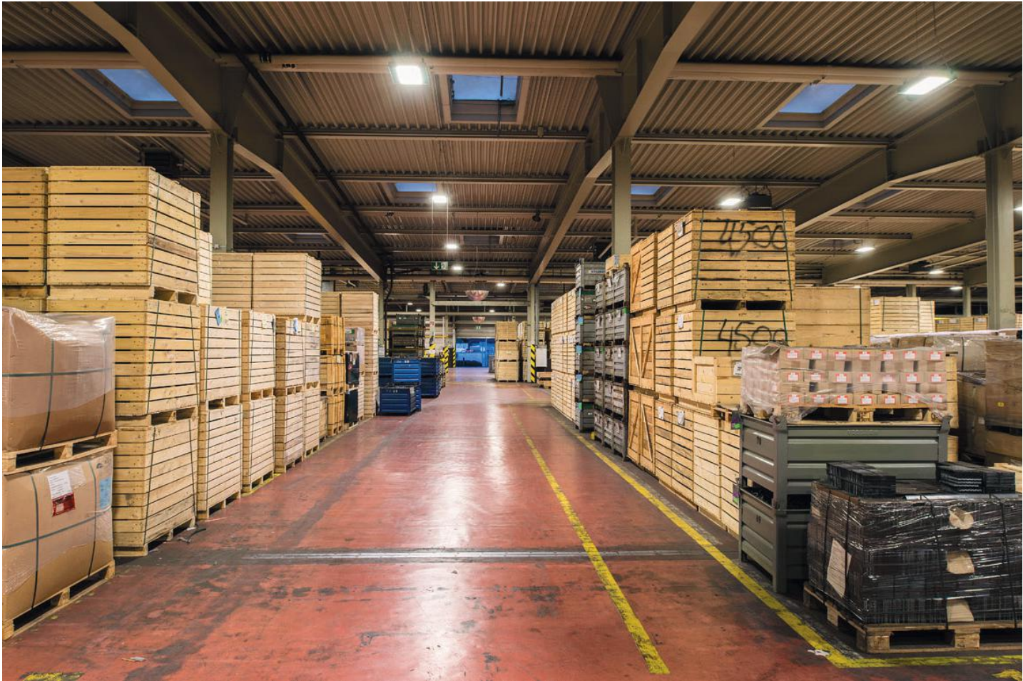
Vossloh warehouse, Luedenscheid, Germany. Luminaire: 176 ©Hoffmeister
